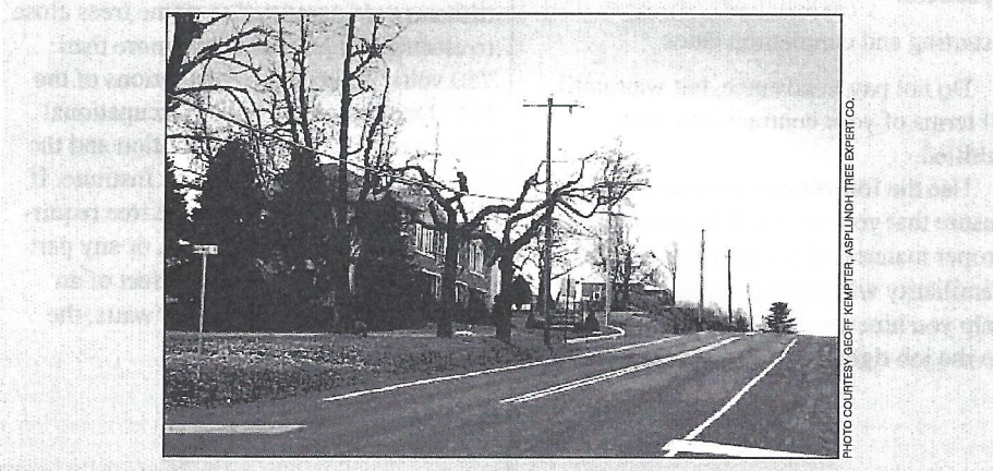
Fig. 6. After directional pruning of the same trees, branches directed away from the wires were retained, instead of removing all of these branches according to previous practices. Much of the regrowth will now occur on those retained branches, without interfering with the wires. Although the shape of the trees appears unnatural in the winter, they will be more normal in appearance when covered with foliage and will be healthier throughout the year.
